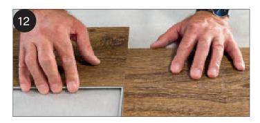
DISASSEMBLING THE SHORT SIDE Disassemble the row by sliding apart the
