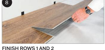
Continue alternating planks on rows 1 and 2 to avoid misalignment. From row 3 onwards, installation does not require alternating rows. Install one row after the other by starting with angling on the long side,
