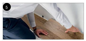
ENGAGE 3<sup>RD</sup> PLANK ON LONG SIDE Take another long plank (3). Repeating the previous step, insert the long side of plank 3 into the long side of plank 2. Then slide plank 3 to your left until the short side is in contact with the short side of plank 1.
