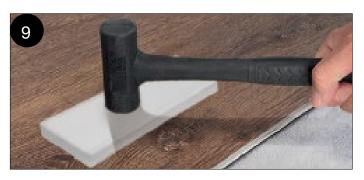
SECURING PLANKS As you go, don't forget to use a rubber mallet on the short sides to secure the locking.
